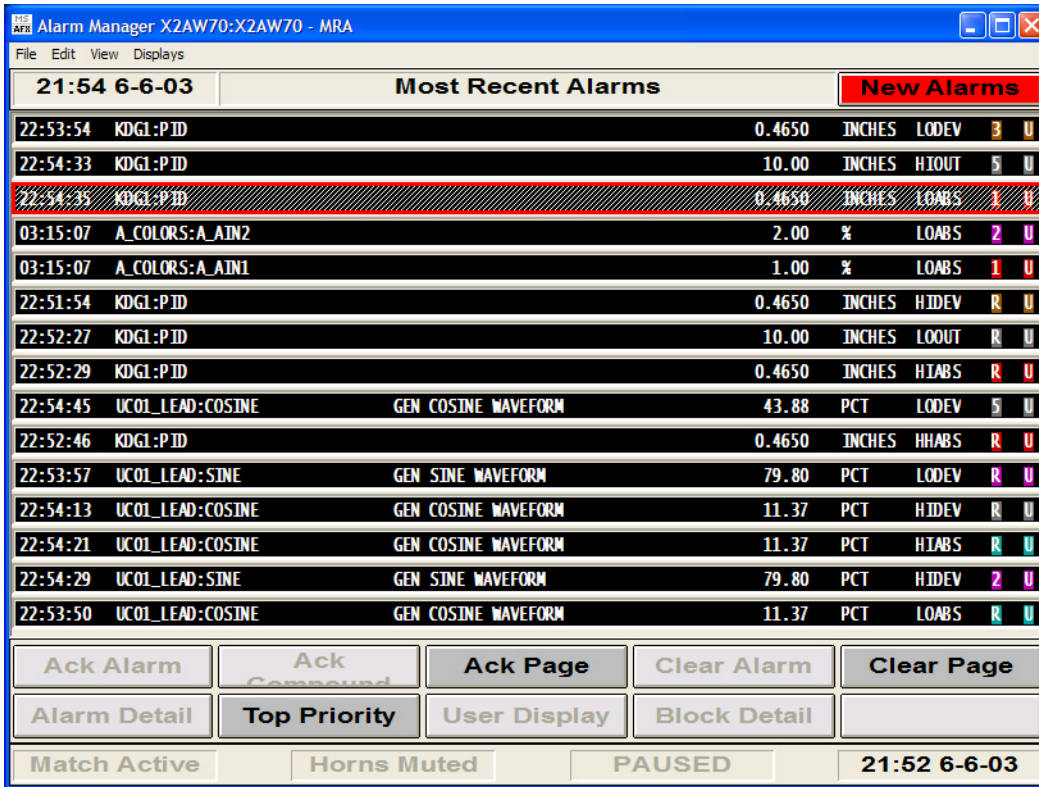
Figure 1. Most Recent Alarms Display
